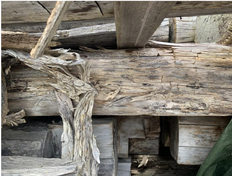
Photo 2: Examples of peeling and flaking on logs
