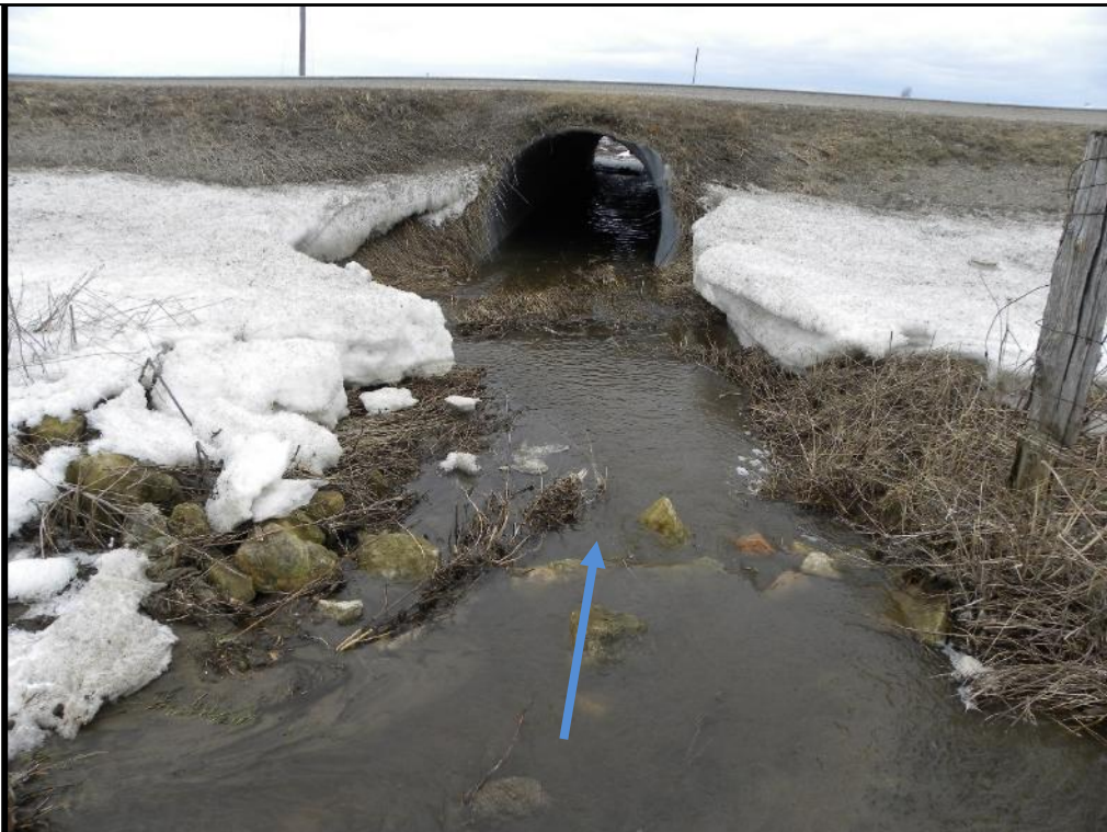
Photo 6: (below) The stream flows under County Road 3 via a culvert into the Brauwer Drain.
