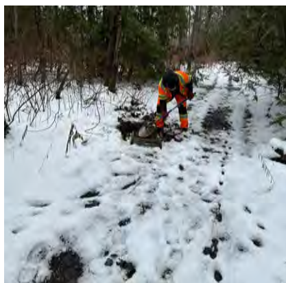
Plate 120: Northeast Area W.I.P. & Test Pit Location/Context; looking north
