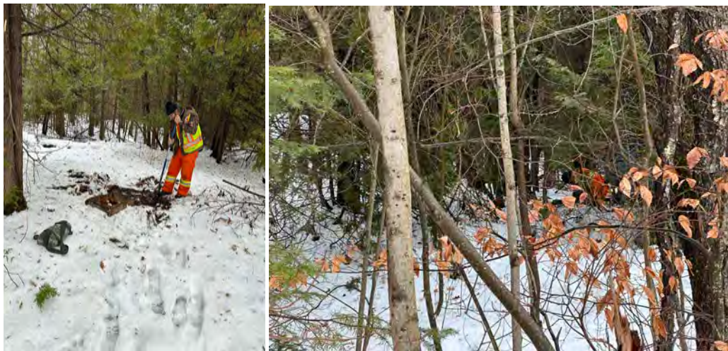
Plates 127-128: North Area W.I.P. & Test Pit Location/Context & bush conditions; looking east & north
