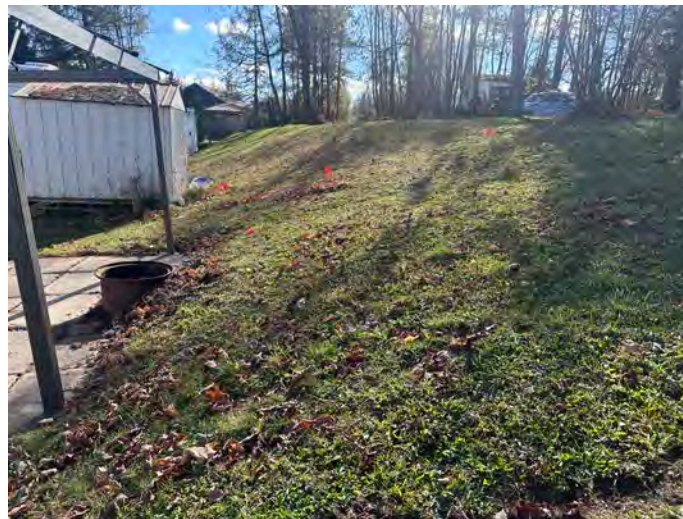
Plate 91: North Central Area Field Conditions with Hydro marked & showing slope; looking southwest
