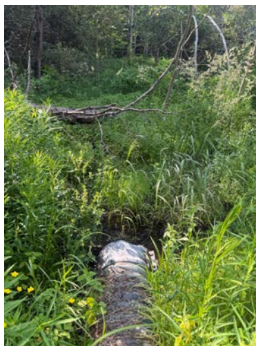
Plate 165: Project Area Field Conditions; looking southeast
