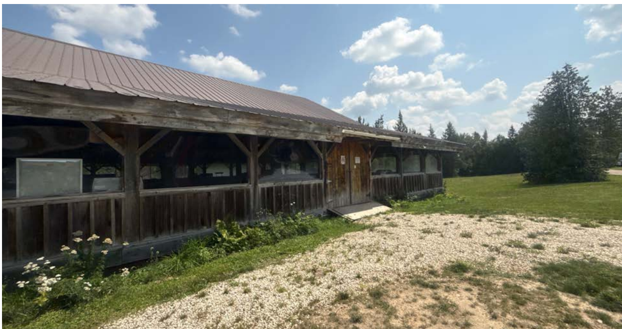
Plate 96: Clubhouse west side; looking southeast
