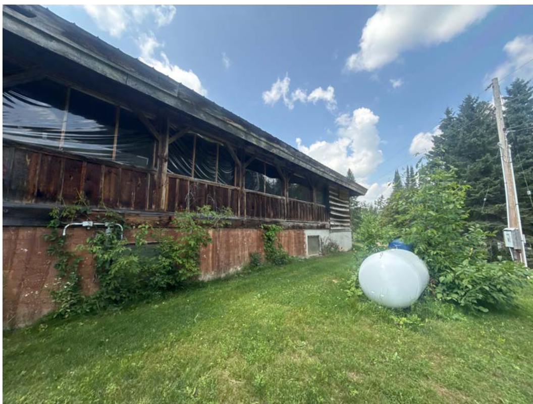
Plate 78: Clubhouse East Side; looking northwest
