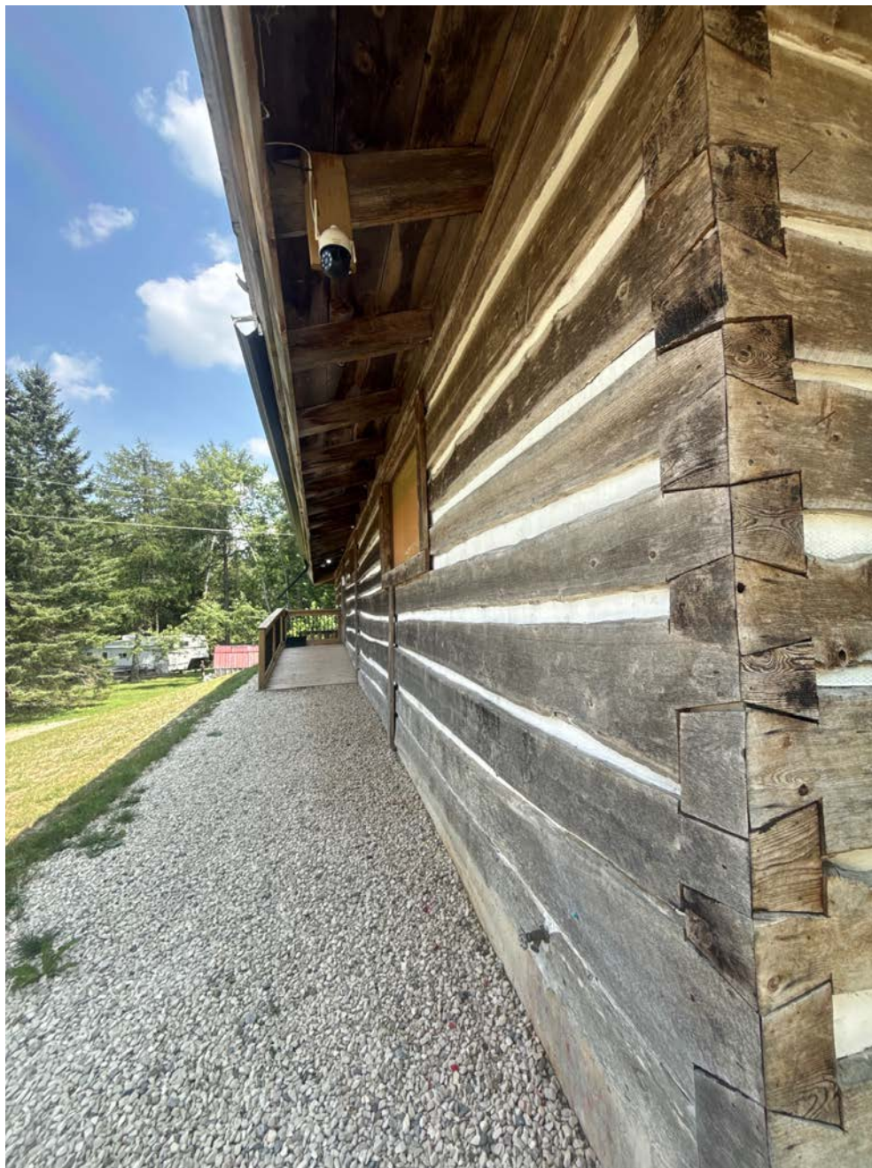
Plate 89: North Addition on north side construction detail; looking west
