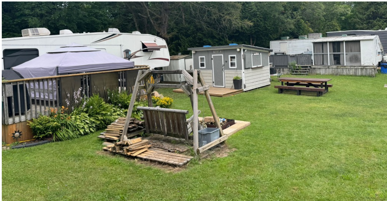
Plate 103: Examples of modified trailers with porches, shed structures & outbuildings
