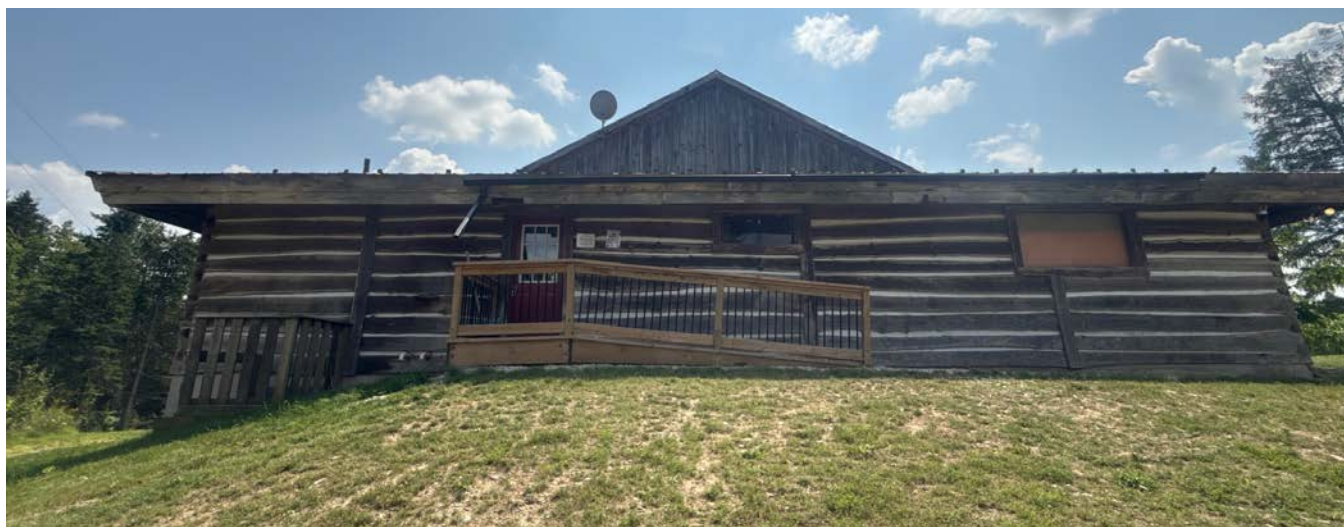
Plate 86: North Addition on north side; looking south
