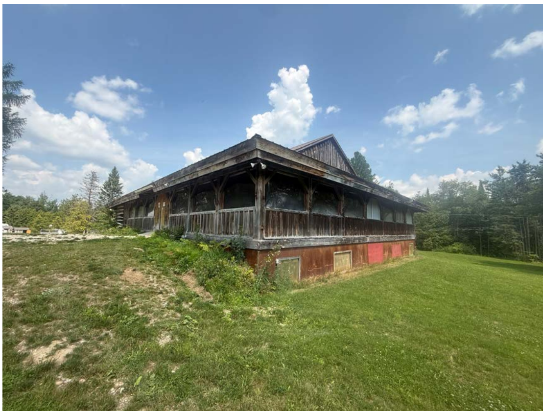
Plate 71: Clubhouse Southwest Corner; looking northeast
