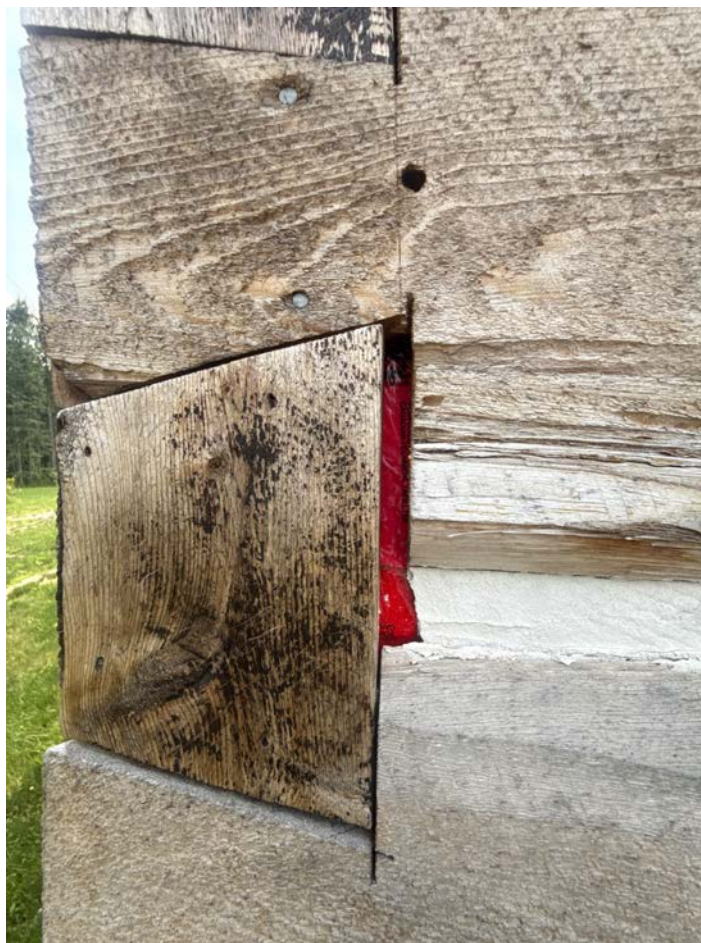
Plate 85: North Addition Construction Detail on north side *NB faux log cabin effect & red plastic vapour barrier under wood & round wire nails; looking south
