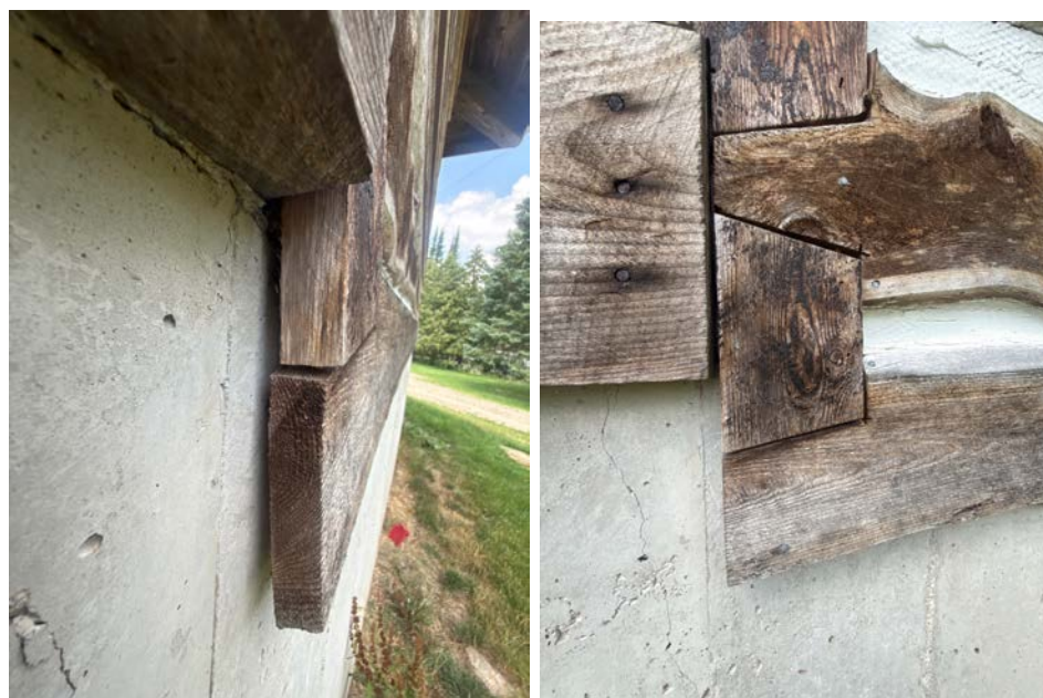
Plates 80-81: North Addition Construction Detail on East Side & Poured Concrete Foundation *NB faux log cabin effect & use of wire (round) nails; looking north & west
