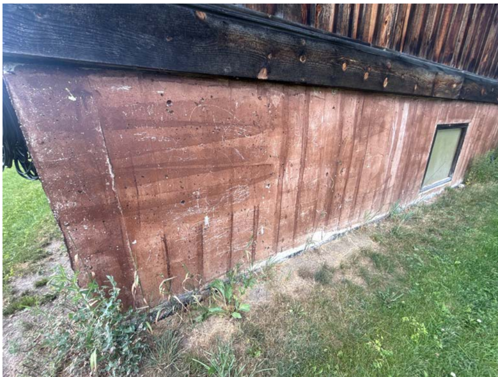
Plate 75: Clubhouse East Side close view of poured concrete foundation; looking northwest
