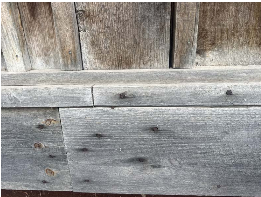
Plate 99: Clubhouse west side construction detail with round wire nails; looking east
