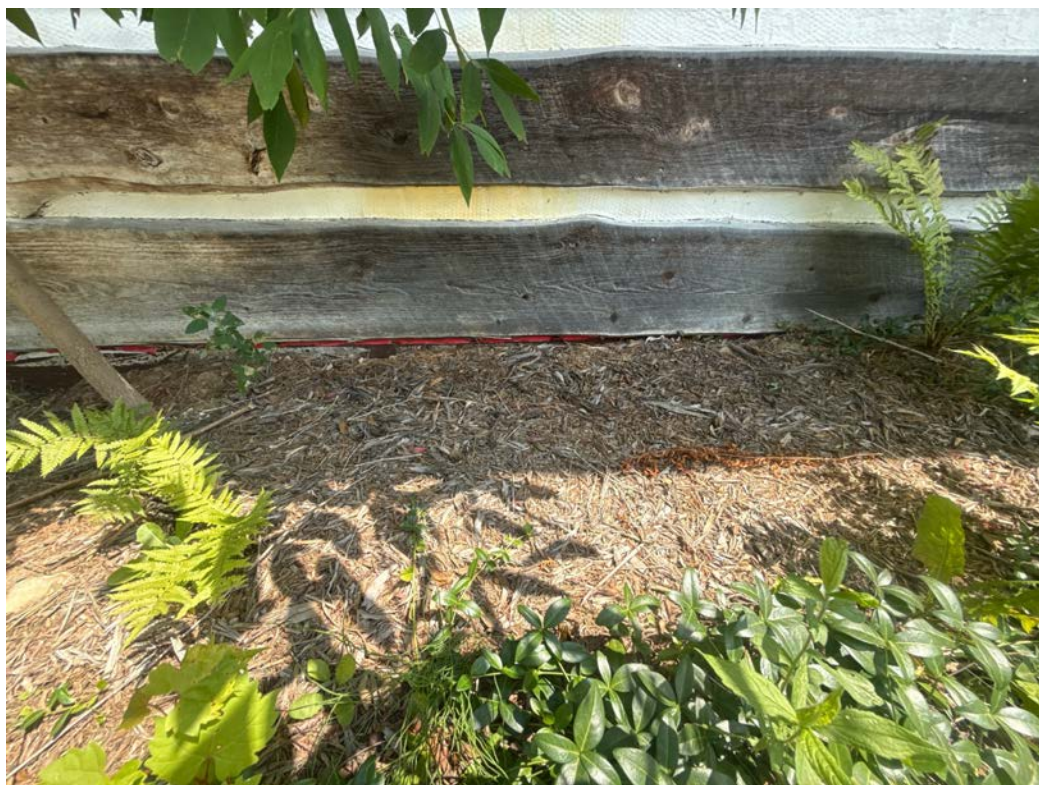
Plate 95: North Addition west side construction detail; looking east
