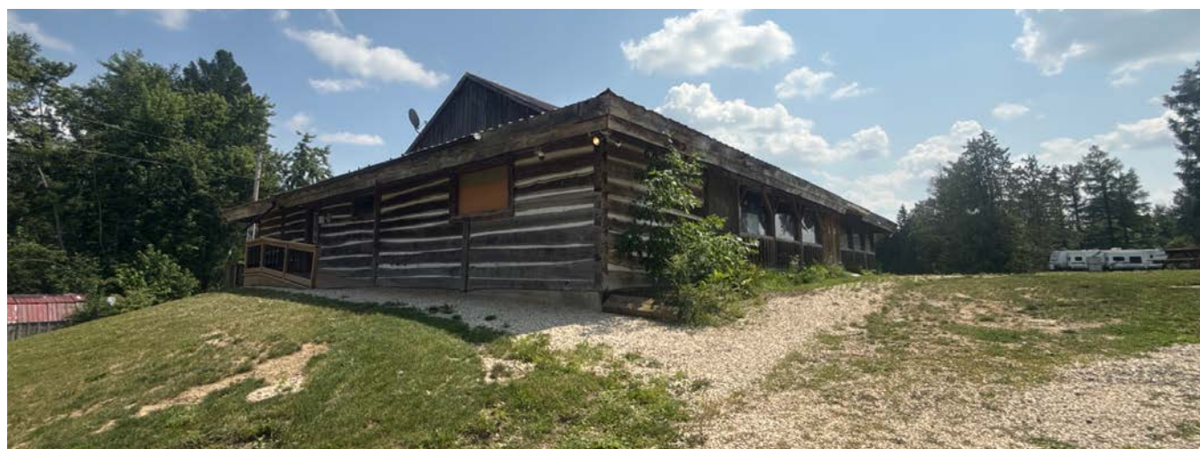
Plate 92: North Addition northwest corner; looking southeast
