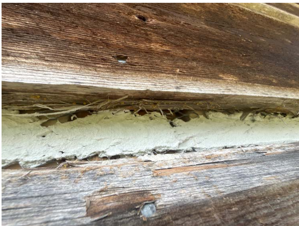
Plate 83: North Addition Construction Detail on north side *NB faux log cabin effect & use of wire mesh; looking south
