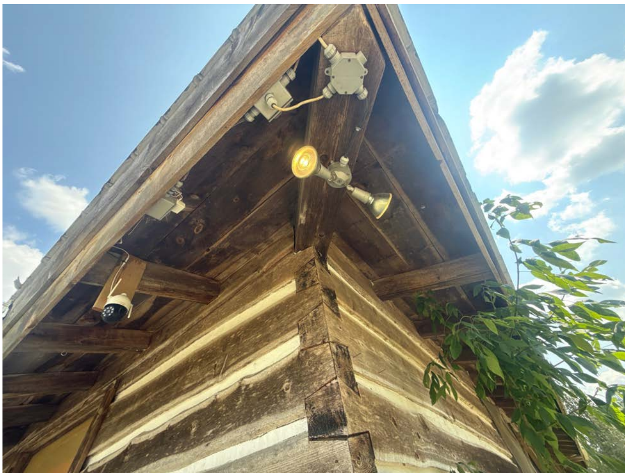
Plate 91: North Addition on northwest corner construction detail; looking southeast
