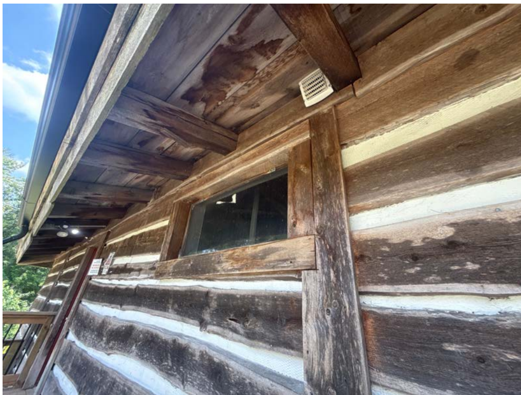
Plate 87: North Addition on north side construction detail; looking southeast
