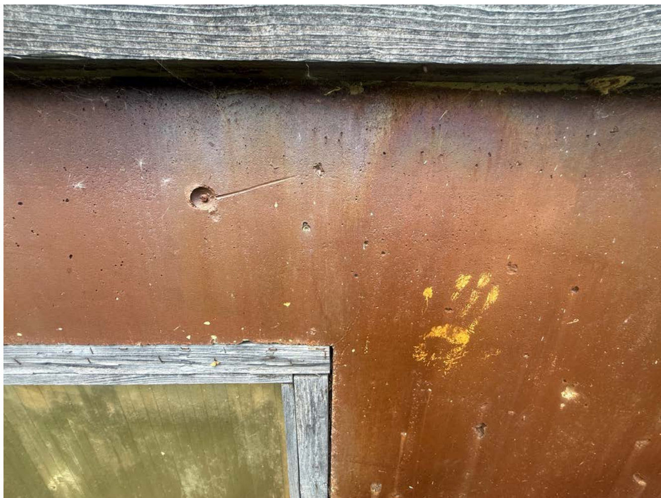
Plate 72: Clubhouse South Side close view of poured concrete foundation; looking north
