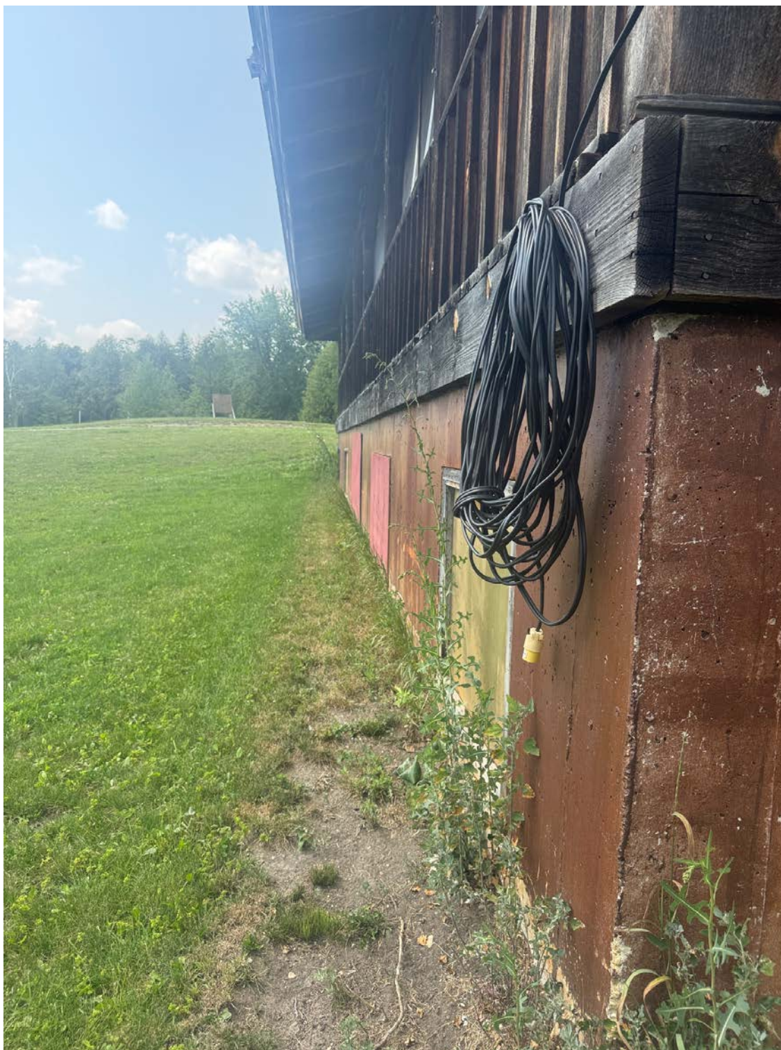
Plate 74: Clubhouse South Side close view of poured concrete foundation; looking west
