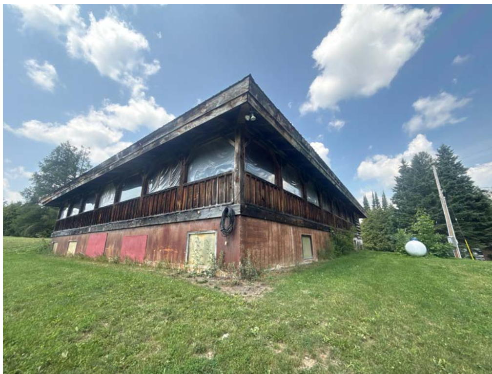
Plate 76: Clubhouse Southeast Corner; looking northwest
