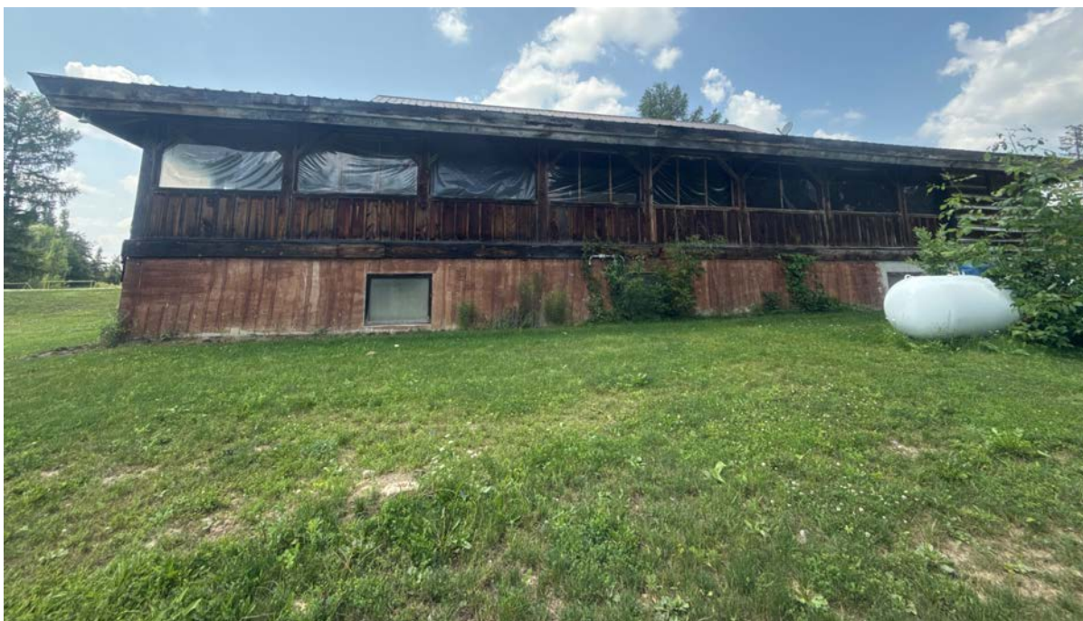
Plate 77: Clubhouse East Side; looking west
