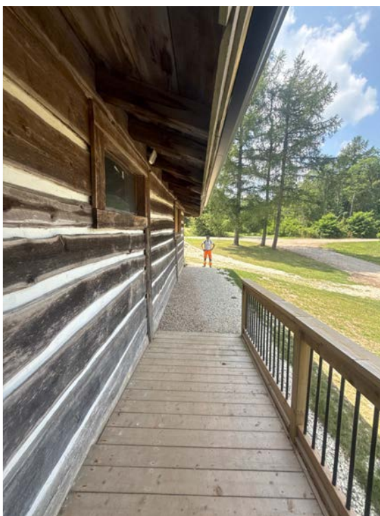
Plate 88: North Addition on north side construction detail; looking east
