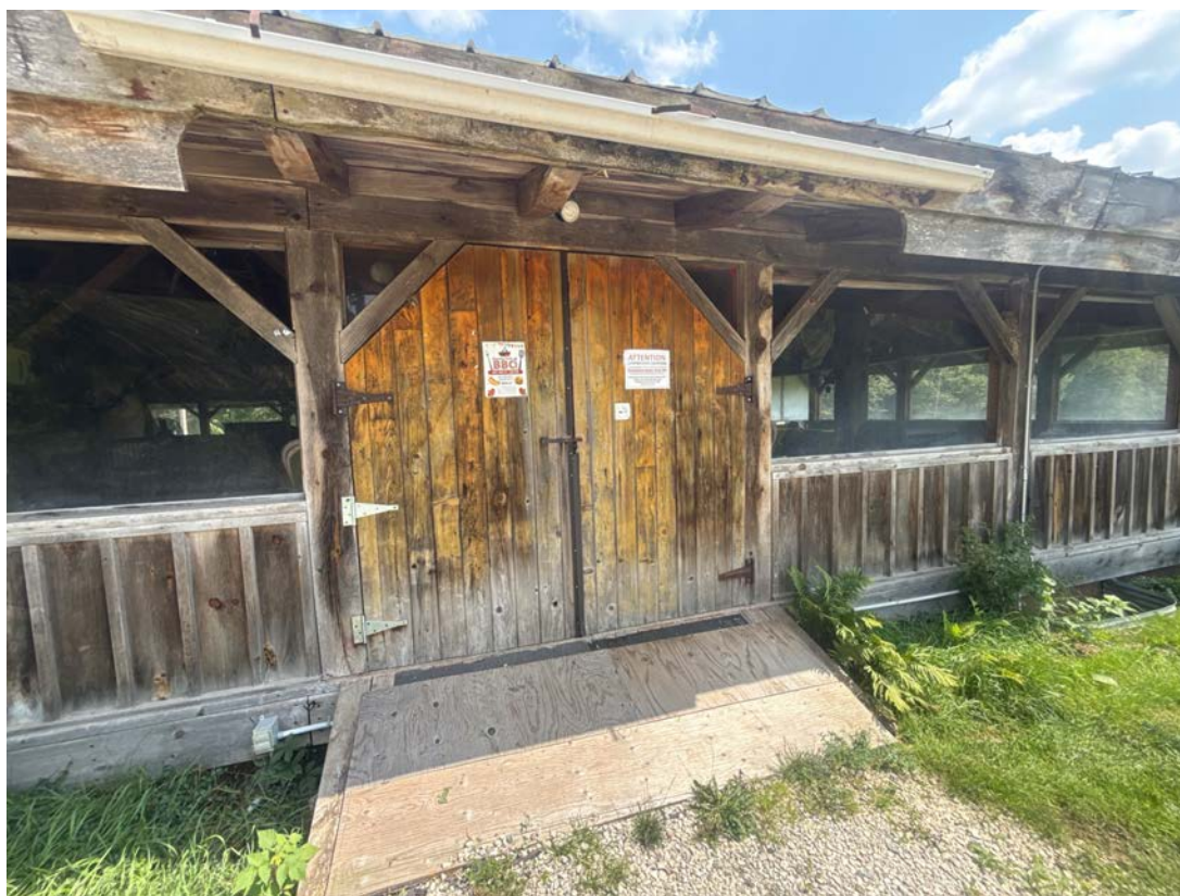
Plate 97: Clubhouse west side; looking southeast
