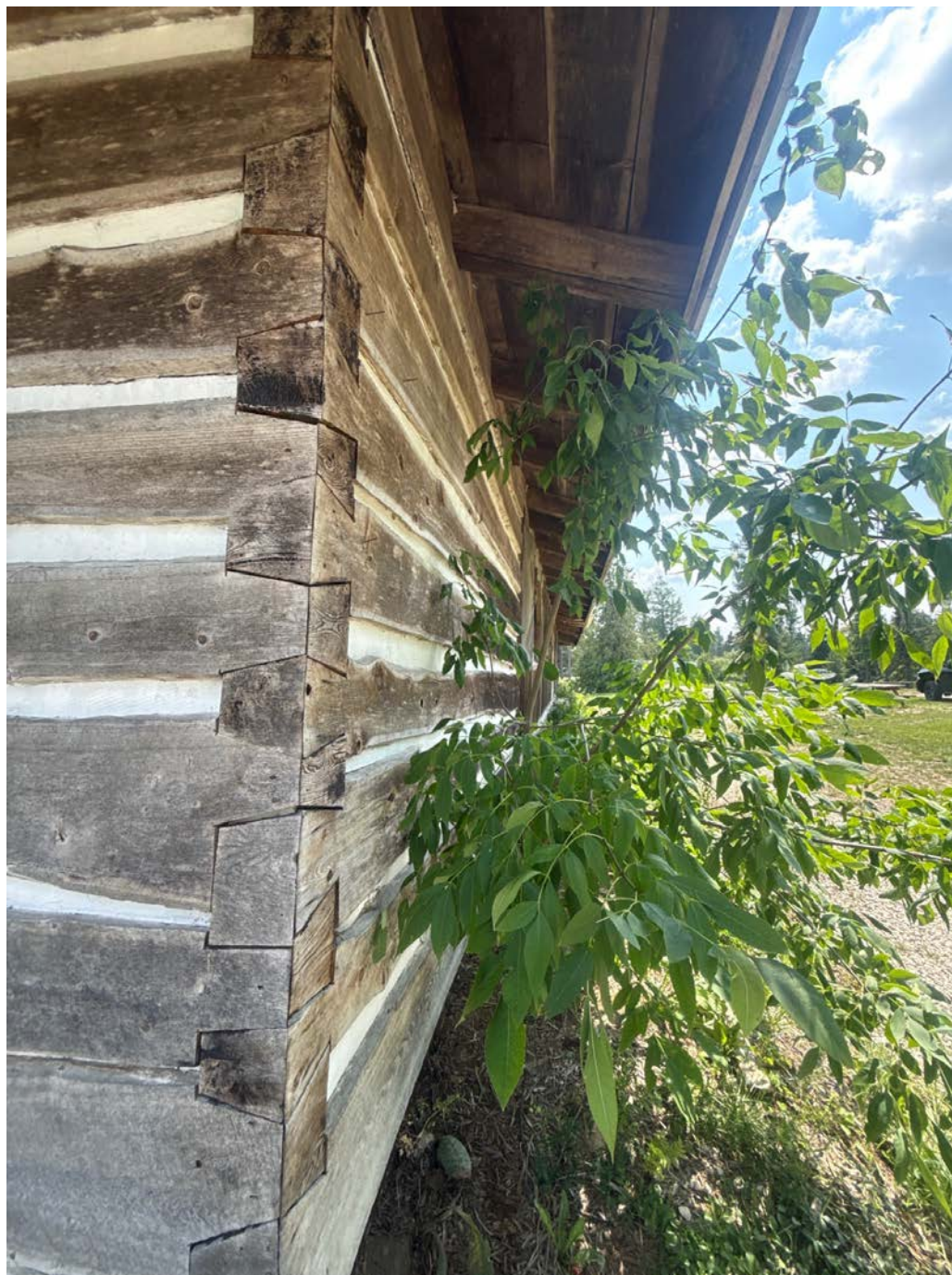
Plate 90: North Addition on north side construction detail; looking south
