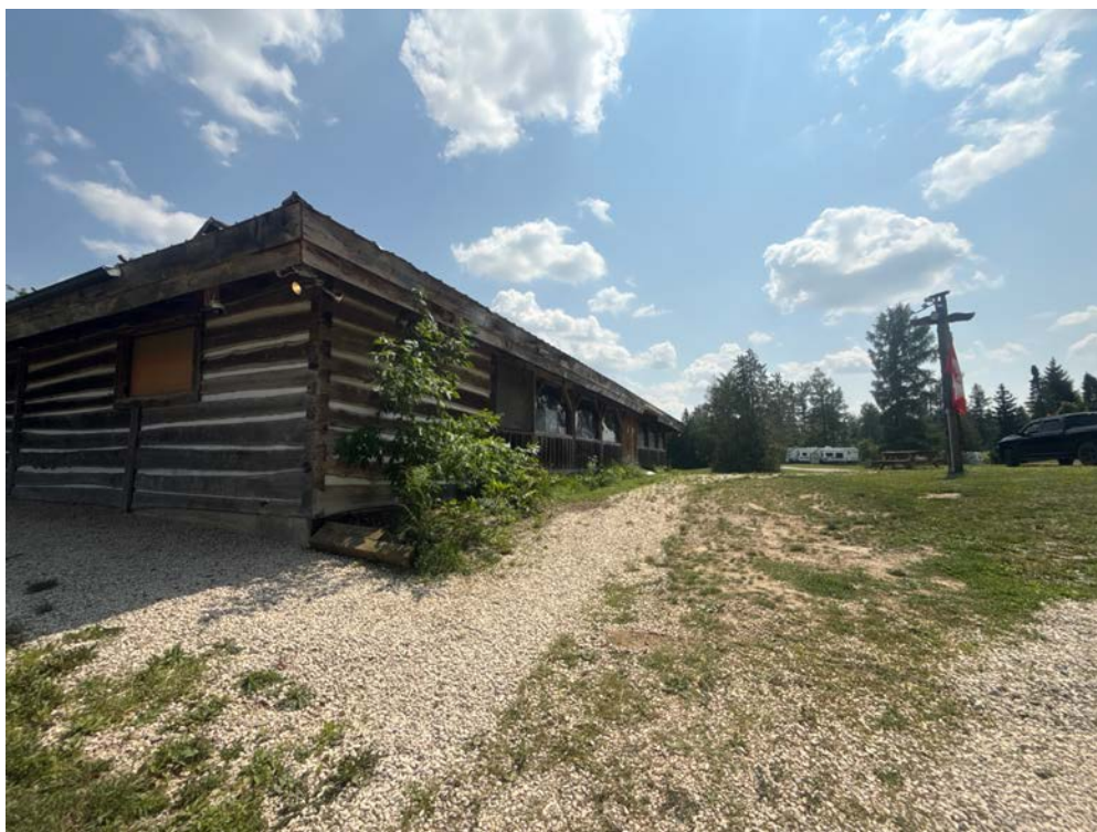
Plate 93: North Addition northwest corner; looking southeast
