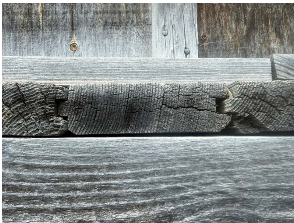
Plate 100: Clubhouse south side construction detail with round wire nails & tongue-and-groove flooring; looking east
