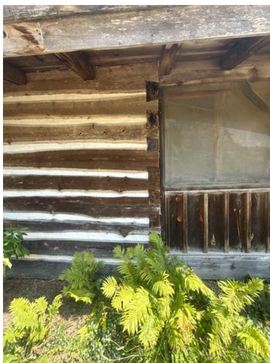
Plate 94: North Addition west side construction detail; looking east
