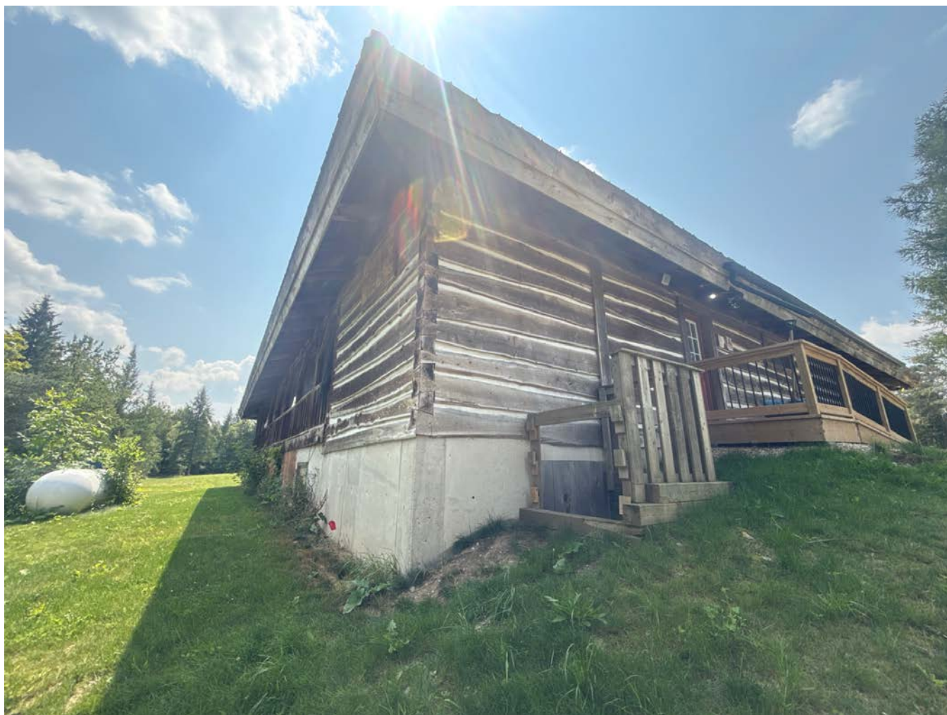
Plate 84: North Addition Construction Detail on north side; looking southwest
