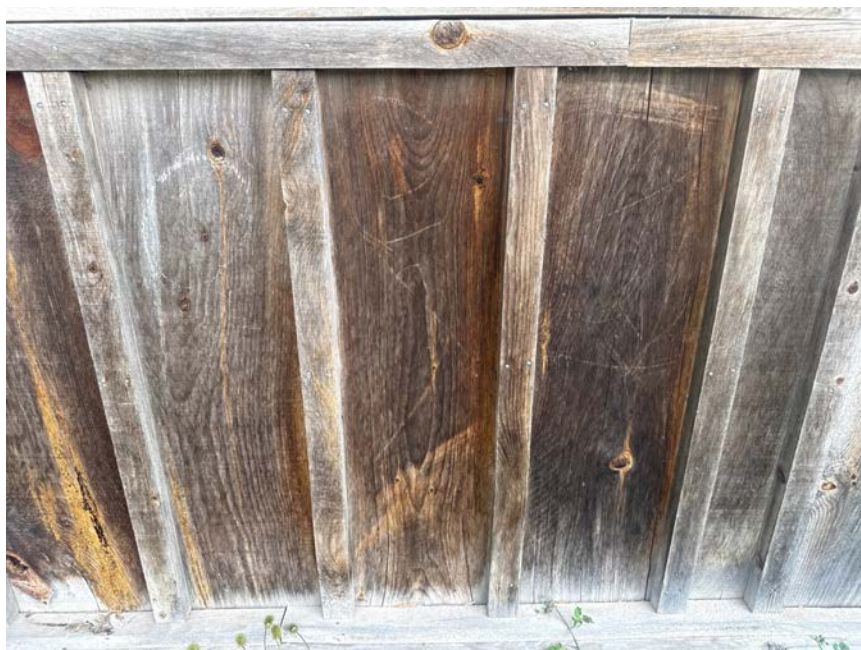
Plate 98: Clubhouse west side construction detail with round wire nails; looking east
