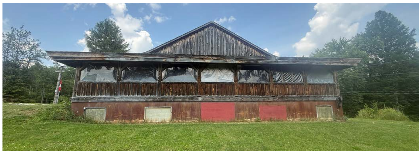
Plate 73: Clubhouse South Side; looking north
