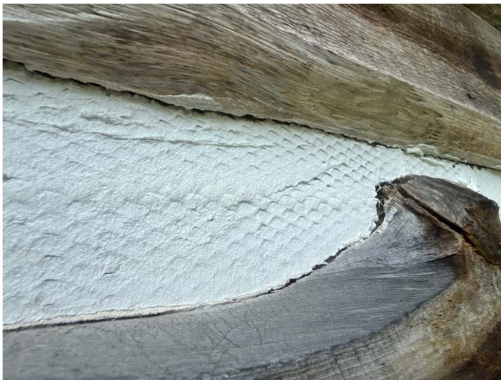
Plate 82: North Addition Construction Detail on north side *NB faux log cabin effect & use of wire mesh; looking southwest
