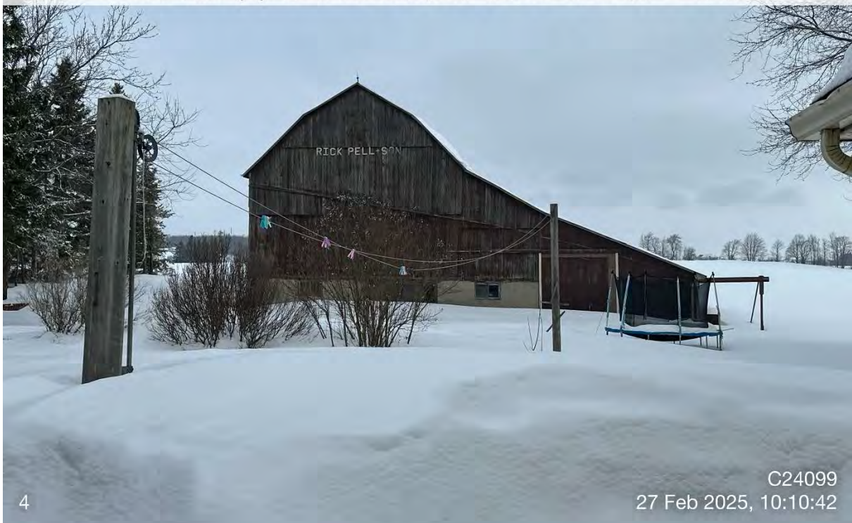
Photo 4: Operation 4 – Wooden bank barn in fair condition.
