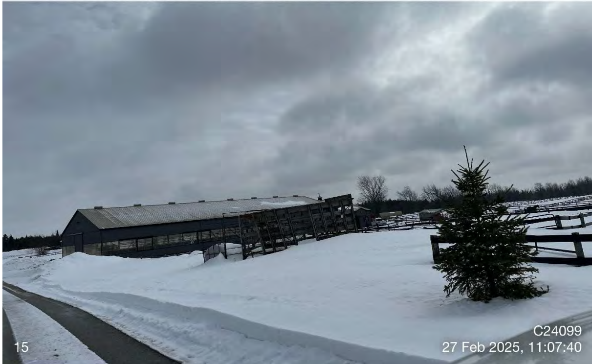
Photo 11: Operation #15 – Indoor riding area, barn with 22 stalls.
