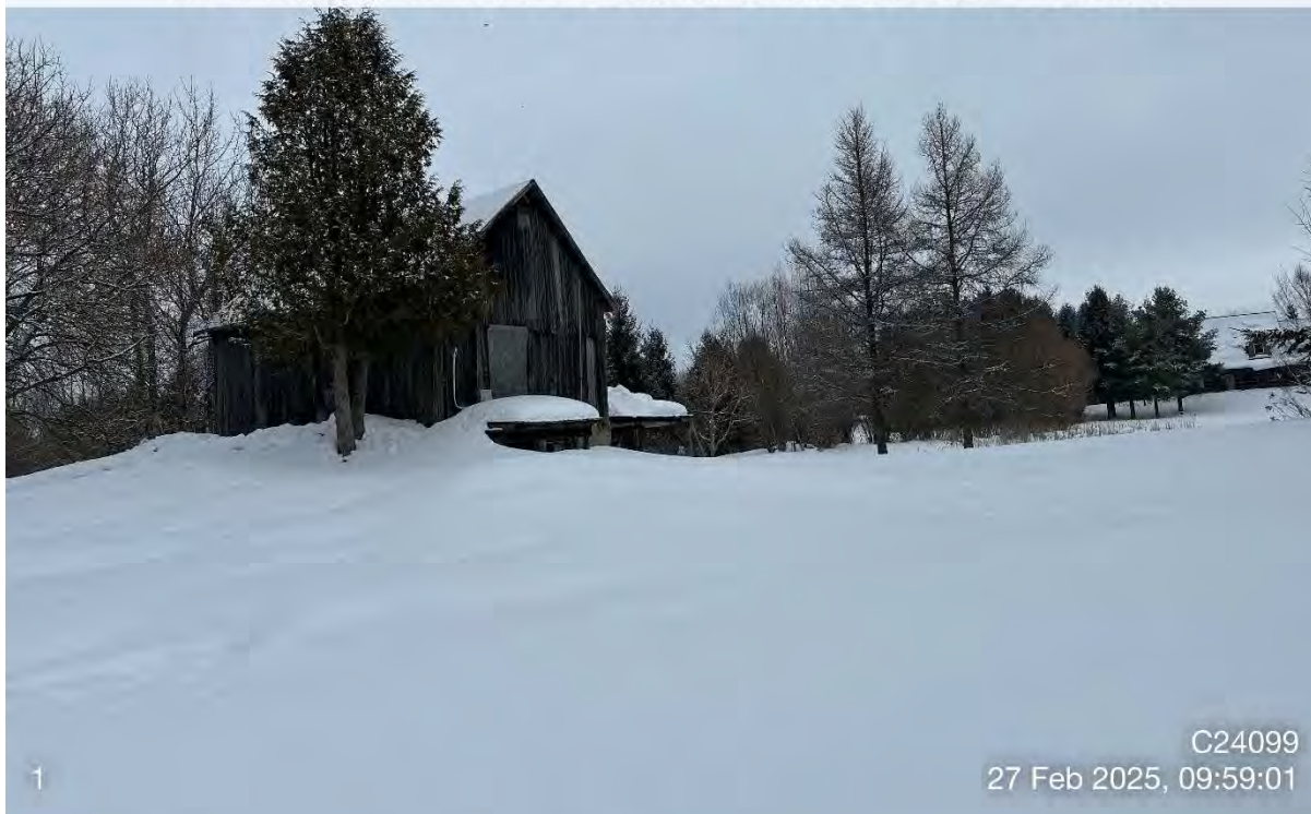
Photo 1: Operation 1 – Small wooden bank barn in poor condition.
