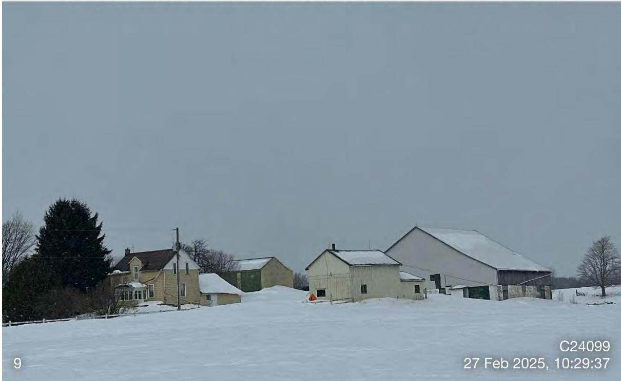
Photo 7: Operation #9 – Barn in fair condition, 2 implement sheds.
