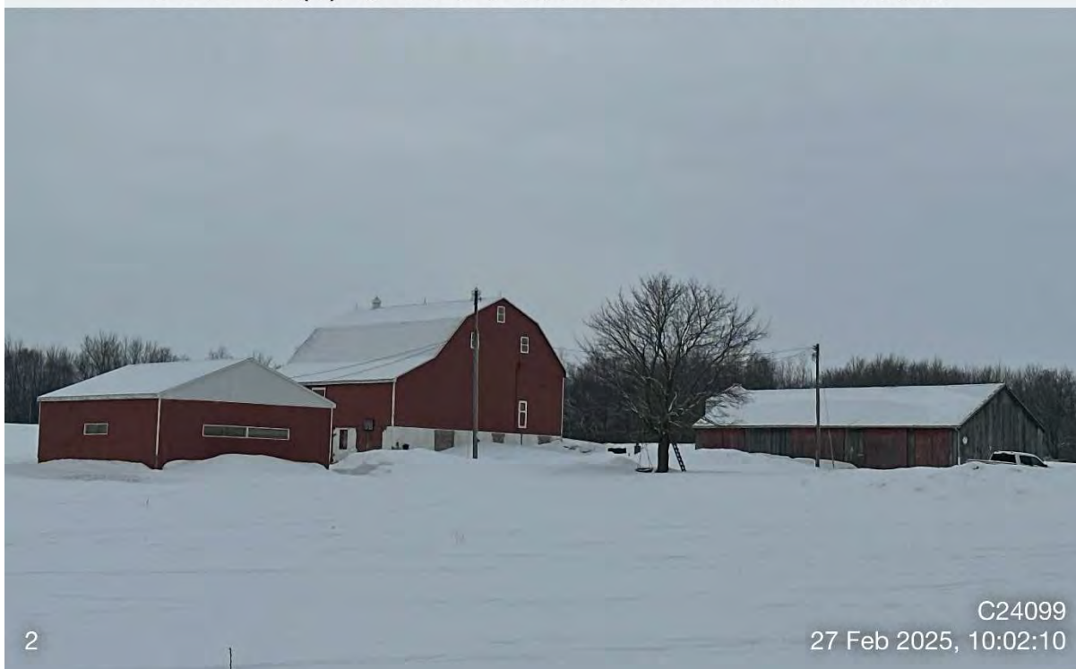
Photo 2: Operation 2 – 2 implement sheds, 1 barn, in good condition.
