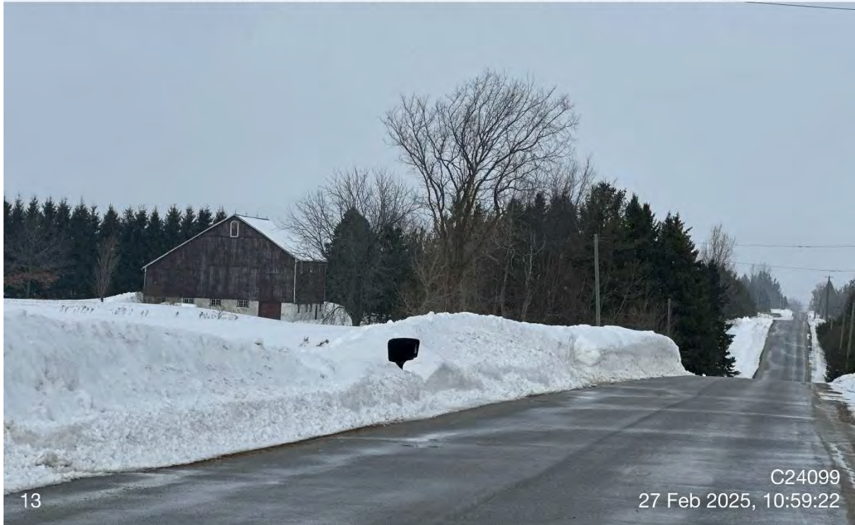
Photo 9: Operation #13 – Wooden bank barn in fair condition.
