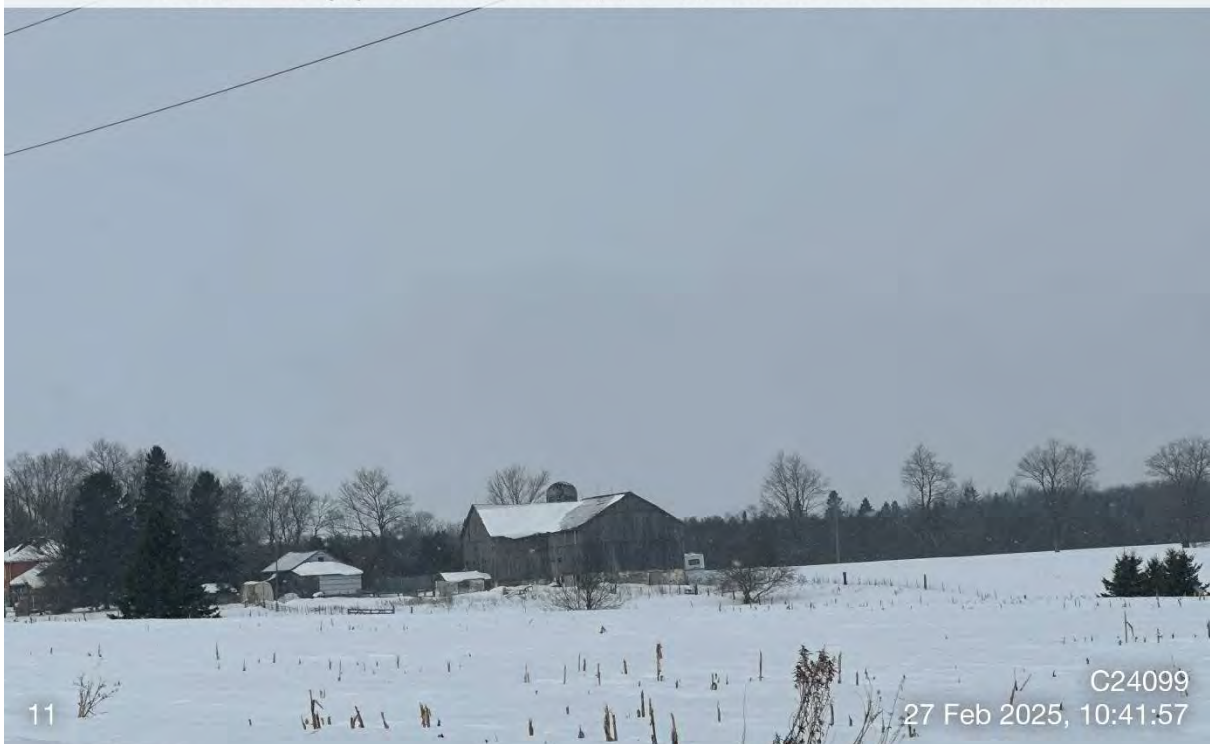
Photo 8: Operation #11 – Wooden bank barn in fair condition, capped silo.
