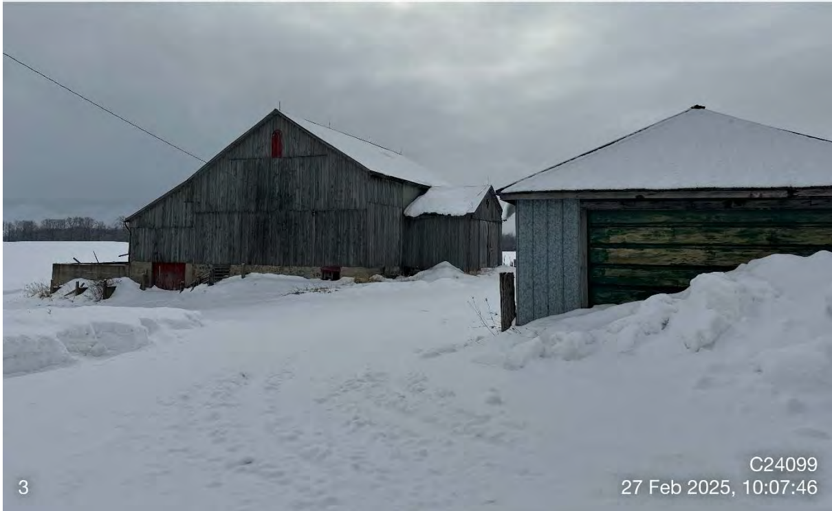
Photo 3: Operation 3 – Wooden bank barn in fair condition, interior in disrepair according to landowner.
