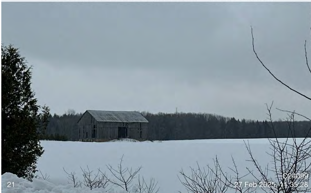
Photo 17: Operation #21 – Wooden bank barn in poor condition, missing more than half of siding.
