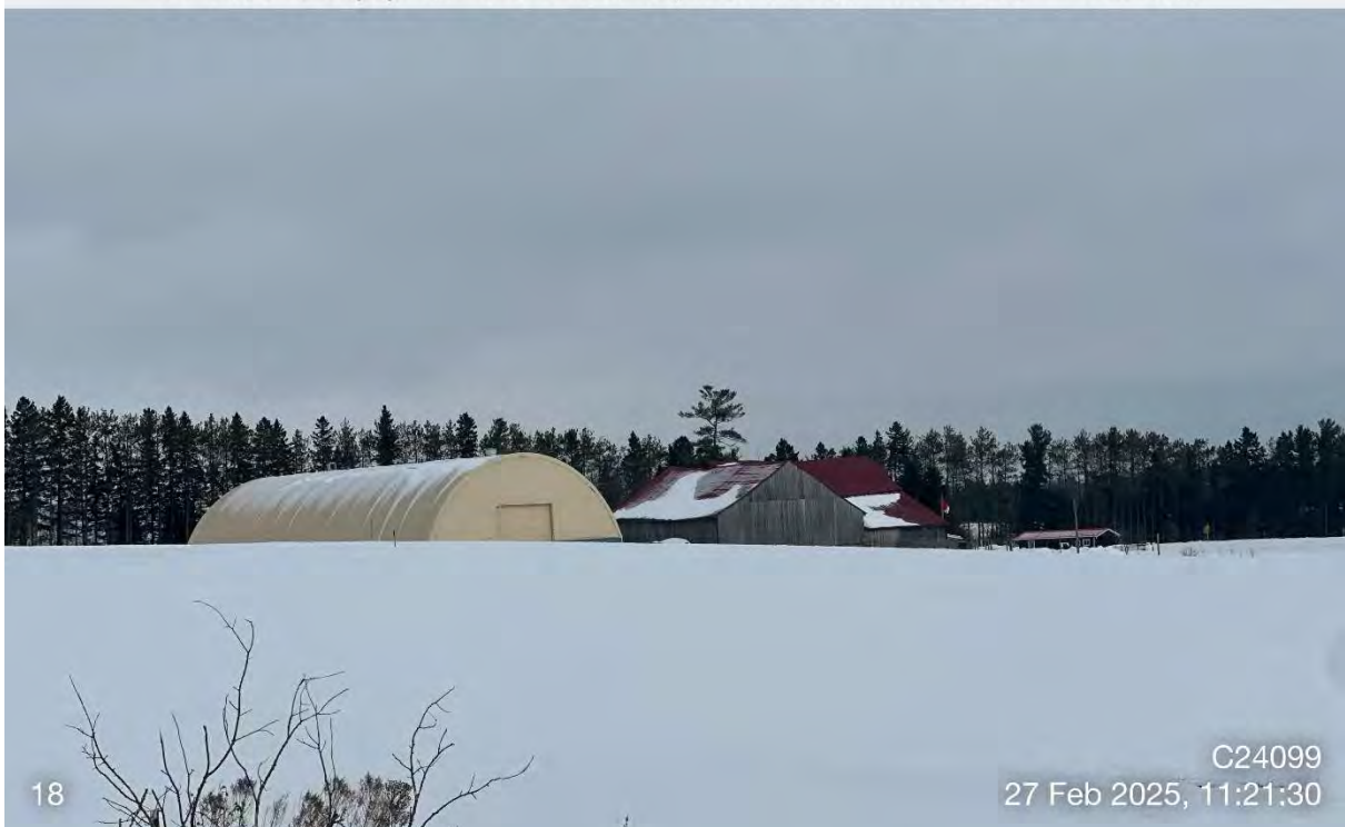
Photo 14: Operation #18 – Large plastic Quonset hut in good contion, wooden bank barn in poor condition with roof partially collapsed.
