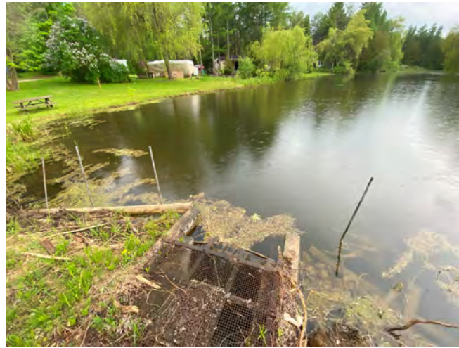
Photo 4: Boyne River Tributary, online pond – pond outlet overflow drop structure (May 22, 2024).
