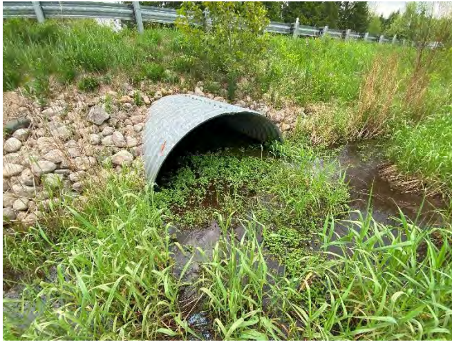
Photo 1: Boyne River Tributary, culvert inlet at 3 rd Line, watercress patches near inlet (May 22, 2024).
