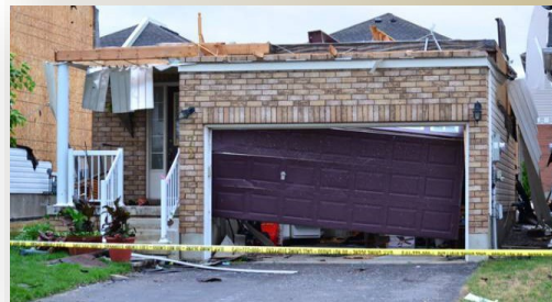
Damage from the Angus Ontario Tornado 2014
