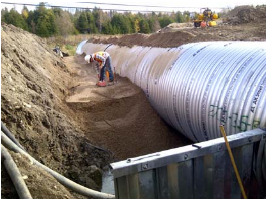
Figures 23 and 24: Compaction Testing of Granular Bedding and Backfill
