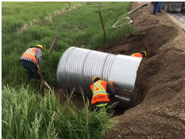
Culvert Extension Dufferin Road 24
