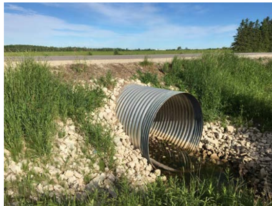
Bosman Drain Culvert – Dufferin Road 12
