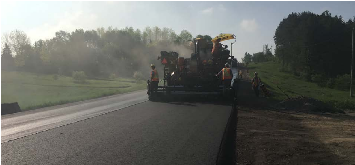
Surface Course Asphalt Dufferin Road 24
