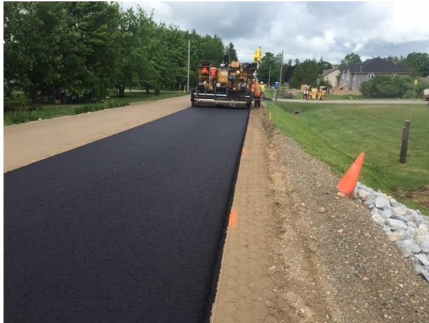
Surface Course Asphalt Dufferin Road 15
