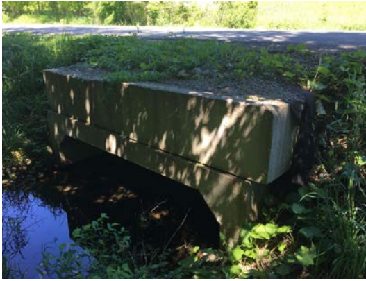
Culvert 004-0909 – Dufferin Road 17
