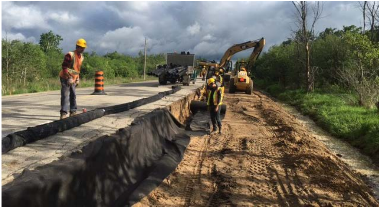
Shoulder Subgrade Preparation and Subdrain Installation Dufferin Road 11
