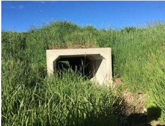
Culvert 032270 – Dufferin Road 5
