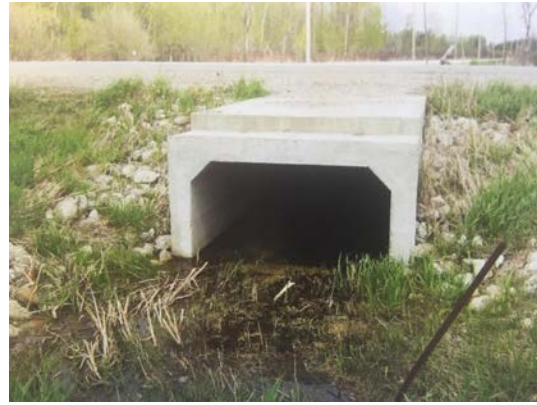
Culvert 032270 – Dufferin Road 5
