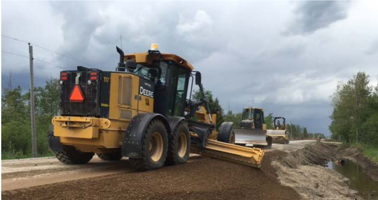
Shoulder Widening Dufferin Road 11
