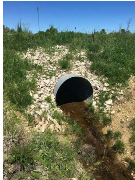
Culvert 784140 Dufferin Road 9
