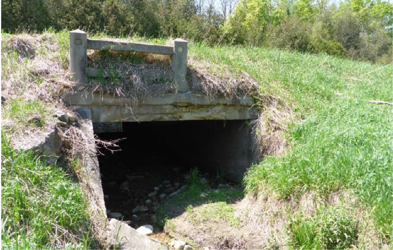
(S1) Culvert (004-2507) – Pre-Construction East Elevation
