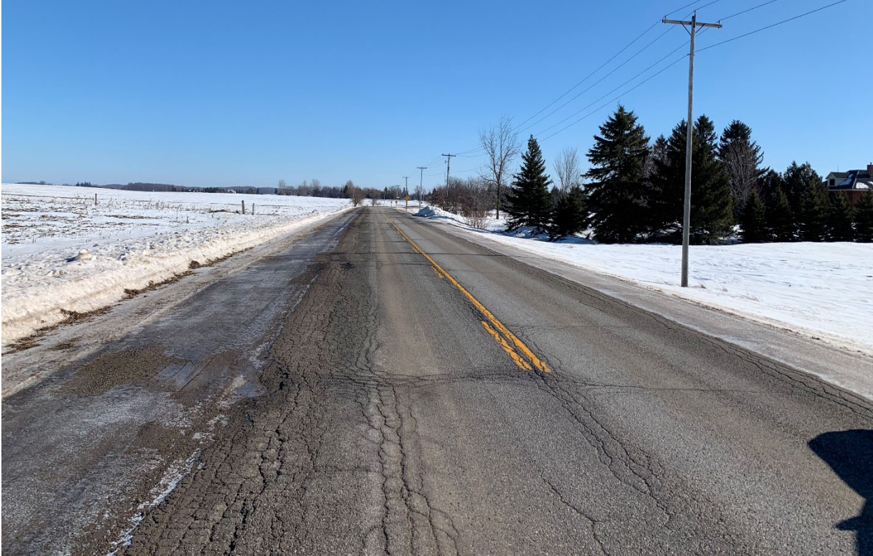
(R2) Dufferin County Road 21 – Pre-Construction Road Condition
