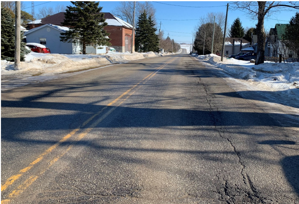
(R2) Dufferin County Road 21 – Pre-Construction Road Condition within Honeywood
