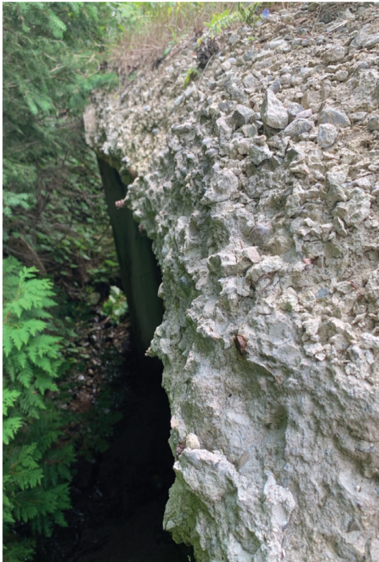
(S3) Culvert (308250XC) –Severe Delamination and Severe Spalling
