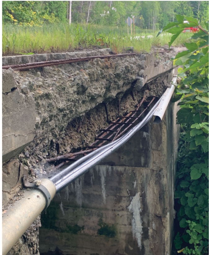
(S3) Culvert (308250XC) –Severe Delamination and Severe Spalling
