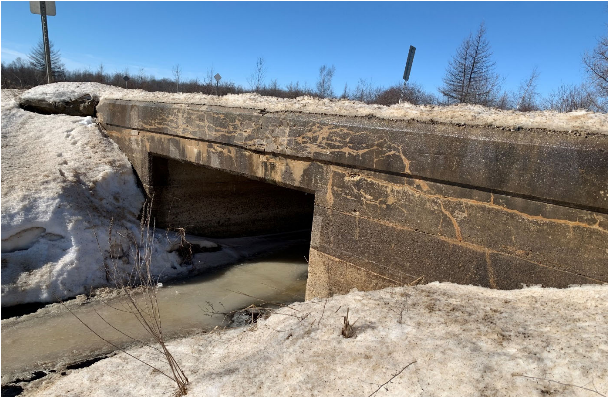
(S4) Culvert 683279CUL – Pre-Construction South Elevation
