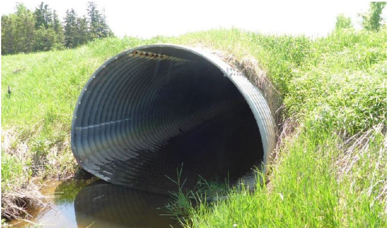
(S2) Culvert (004-2508) – Pre-Construction East Elevation
