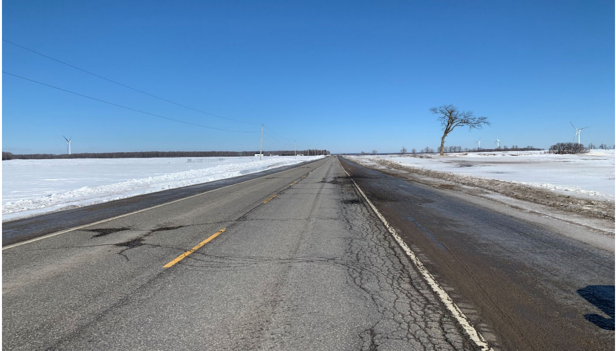
(R1) Dufferin County Road 124 – Pre-Construction Road Condition
