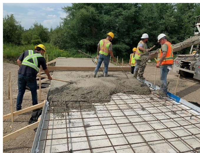
Distribution slab on Culvert 683279
