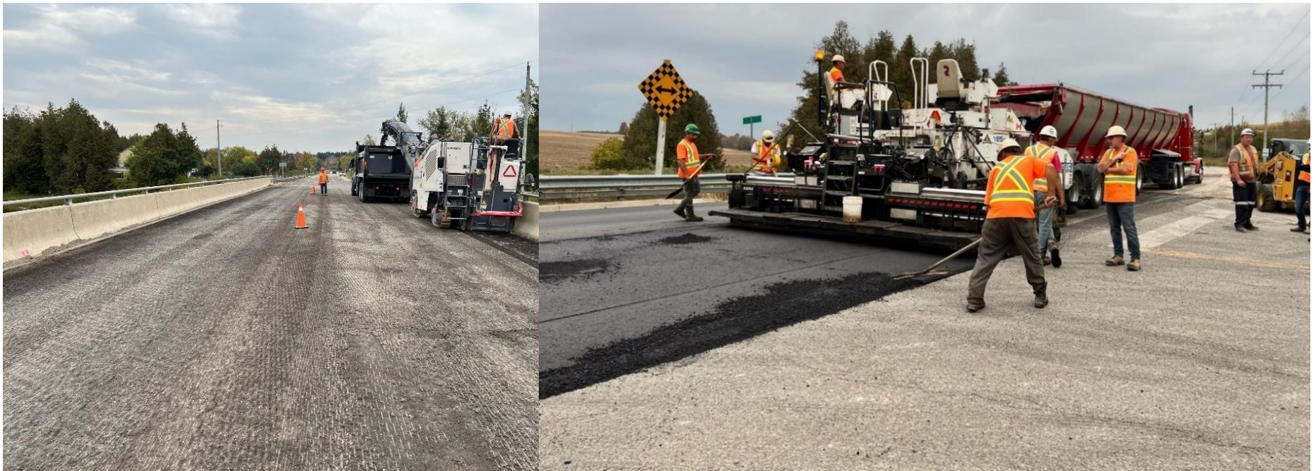
Milling and Resurfacing of Black Bridge (004-0063)
