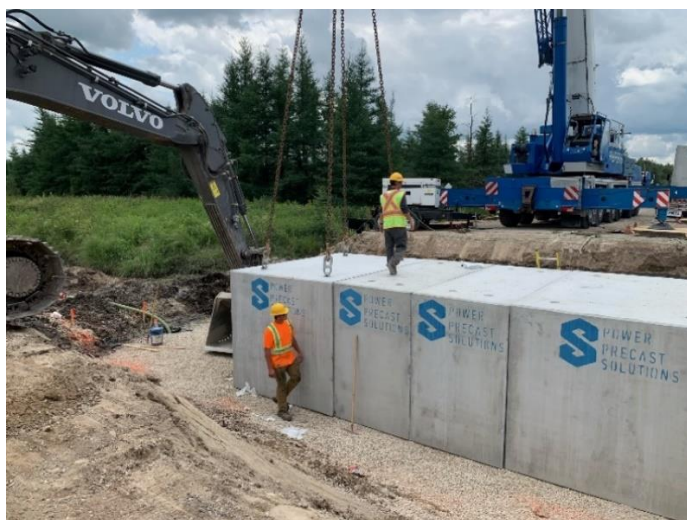
Installation of Precast Concrete Culvert 683279
