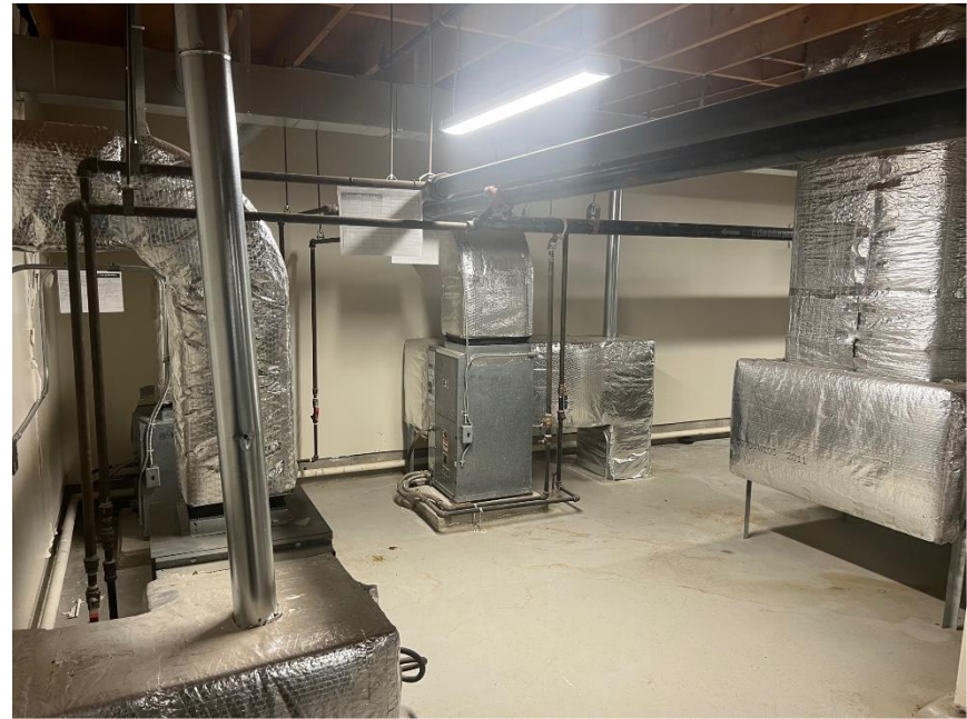
Courthouse heating, ventilation, and air conditioning upgrades
