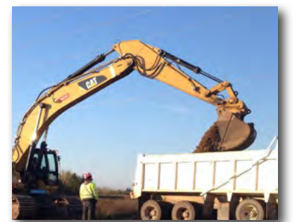
Reconstruction of County Road 21
