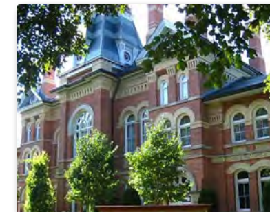
Heritage Restoration of County Courtroom 204
