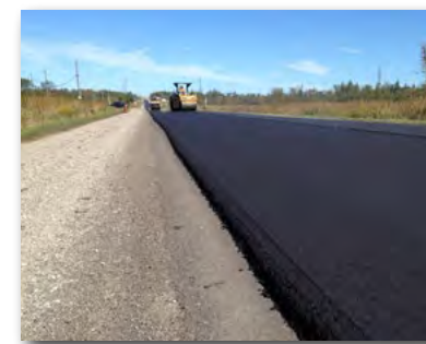
Reconstruction of County Road 109
