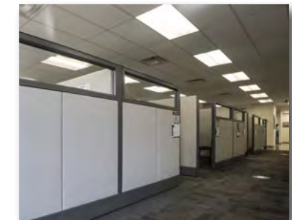
Building Condition Assessment
