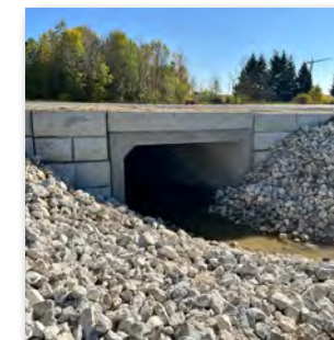
Biennial Assessment of Bridge and Large Culvert Structures
