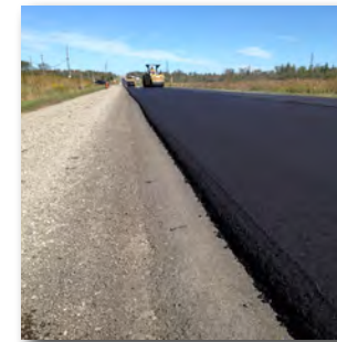
Capital Road and Large Structure Construction/ Rehabilitation
