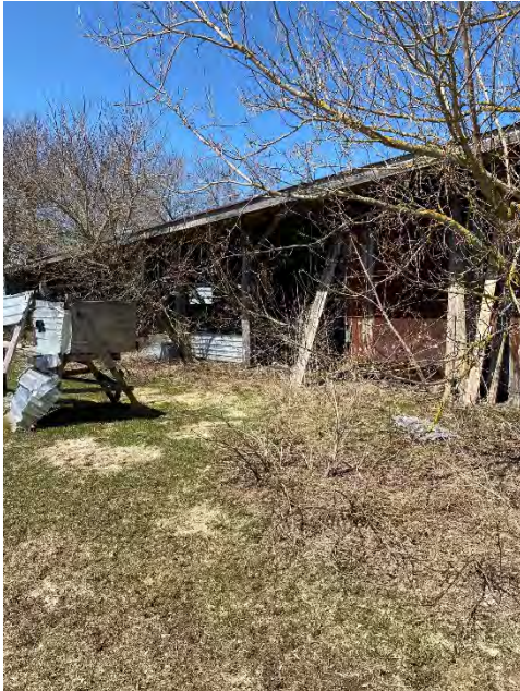
Run in Barn on site (Paintball/Airsoft Scrap pictured right)
