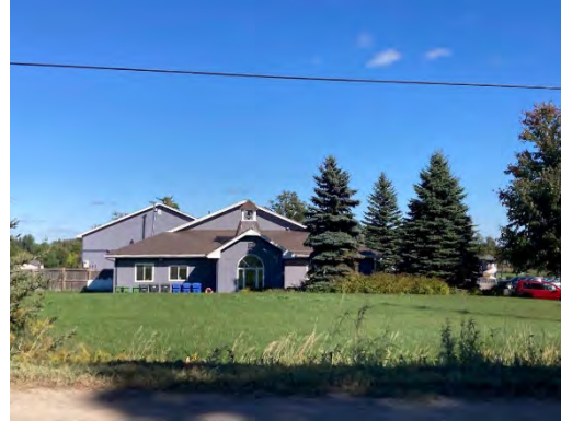
Image 7: View of Maples Academy Private School building on the 2 nd line
