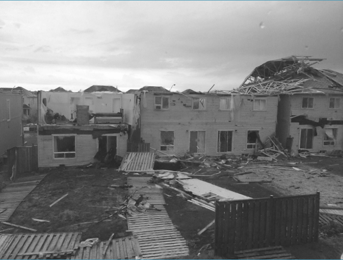
Tornado Damage – Angus, Ontario – 2014
