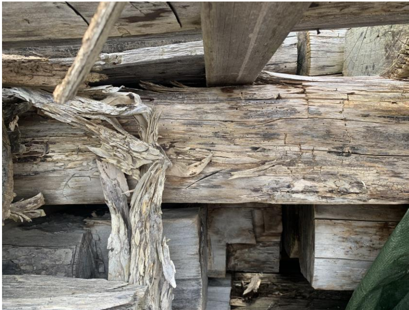
Photo 2: Examples of peeling and flaking on logs
